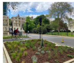
Parking and kerbside
