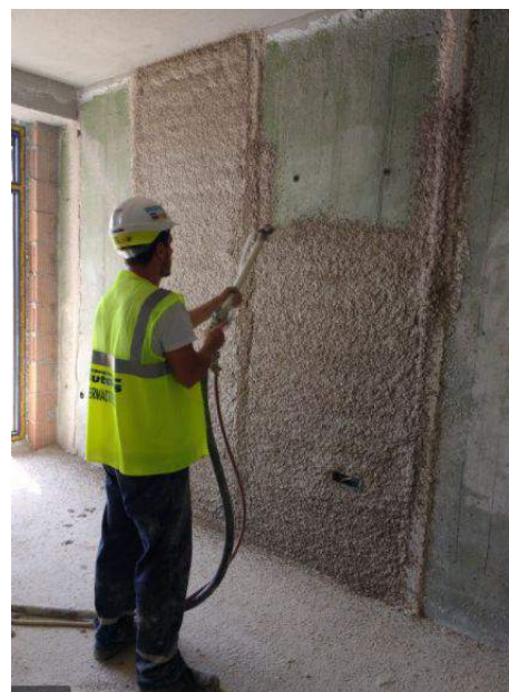
Wet applied insulating plaster
