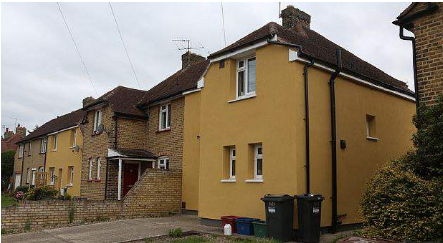
The above external wall insulation and window improvement scheme by Hounslow Council has helped making these homes much more efficient and comfortable. In the future, these schemes should ideally be offered and extended to interested leaseholders, which will take time in terms of communication at the outset of the project.
